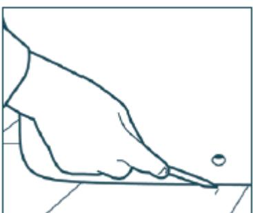
Toilet frame is marked on the floor. Side installation hole axis is also marked on the floor.
