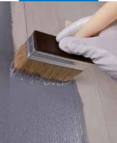
Application of Eco Prim Grip Plus on concrete by brush
