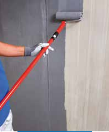
Application of Eco Prim Grip Plus on concrete by roller
